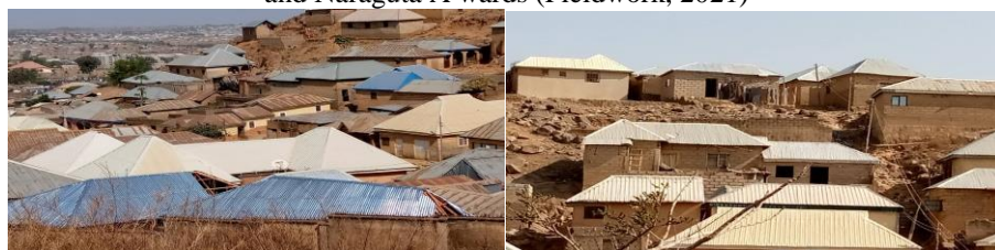
Plate 2 Fragmentation of plots, illegal and unplanned development, poor and unmotorable access roads, absence of pipe borne water and sanitation, electricity and building congestion in emerging segregated residential settlements in Kabong and Naraguta A wards (Fieldwork, 2021)
