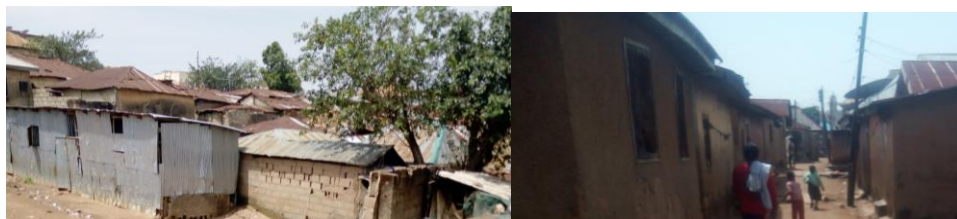
Plate 1 Fragmentation of plots, illegal and unplanned development, poor and unmotorable access roads, absence of water and sanitation, erratic electricity, building congestion in the older segregated residential settlements in Kabong and Naraguta A wards (Fieldwork, 2021)
